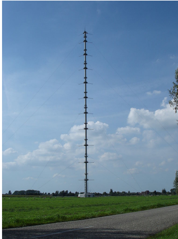
Figure 2 The Cabauw tower.
